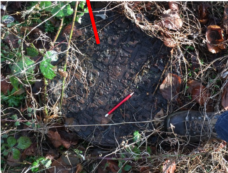
Manhole observed during Site Visit 31/1/18
